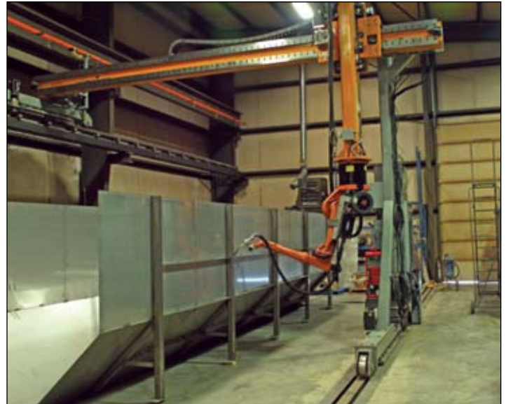
NINE AXES OF PERFORMANCE — The newly-completed gantry robot performs its first welds on a piece of scrap stainless steel in July. It now welds 10-foot by 32-foot stainless steel clarifiers (wastewater) tanks used in VanAire's Dissolved Air Flotation system. (Photo courtesy of VanAire, Inc.)
