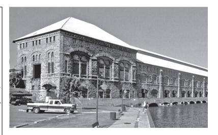
**Utility System Infrastructure**: The entire building interior needs to be remodeled. The mechanical and electrical systems are old and inefficient. The space configuration does not meet the current needs. The building does not meet ADA standards for plumbing or multi-floor access. The building is listed with the National Historic Civil Engineering Landmarks.
